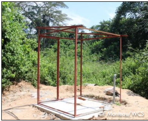
Construction of six community long-drop toilets in Bomassa and Bon-Coin.
